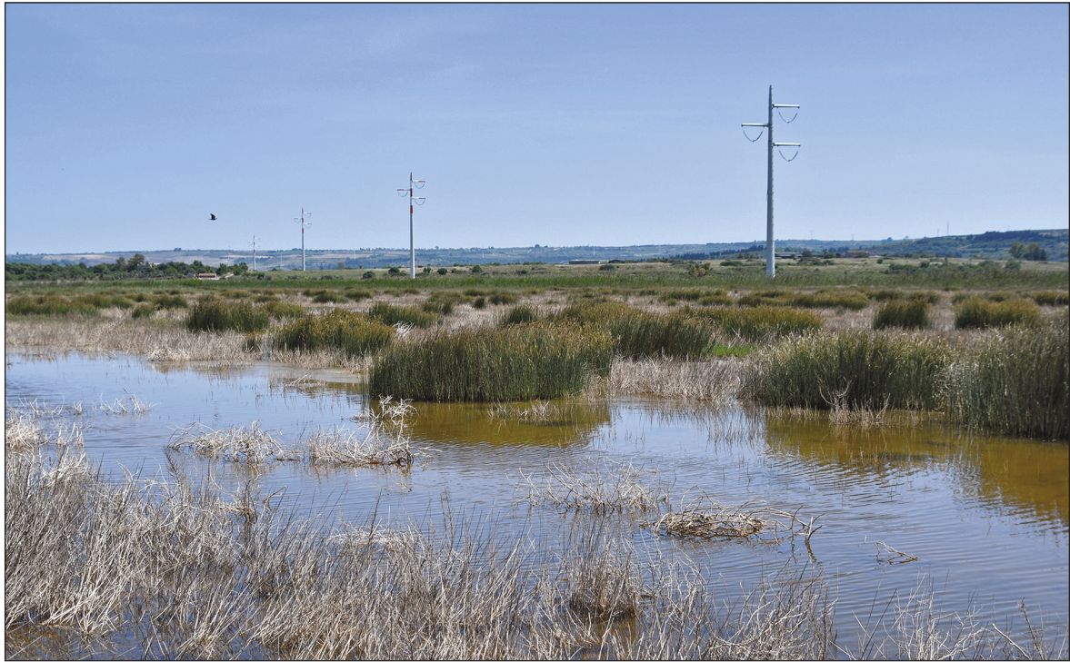
Figure 1. The landscape impact produced by the power line will be irremediable and unmitigated. Photo shows the crossing of the Lentini marsh by the power line that is still without the conductors (May 14, 2022).
