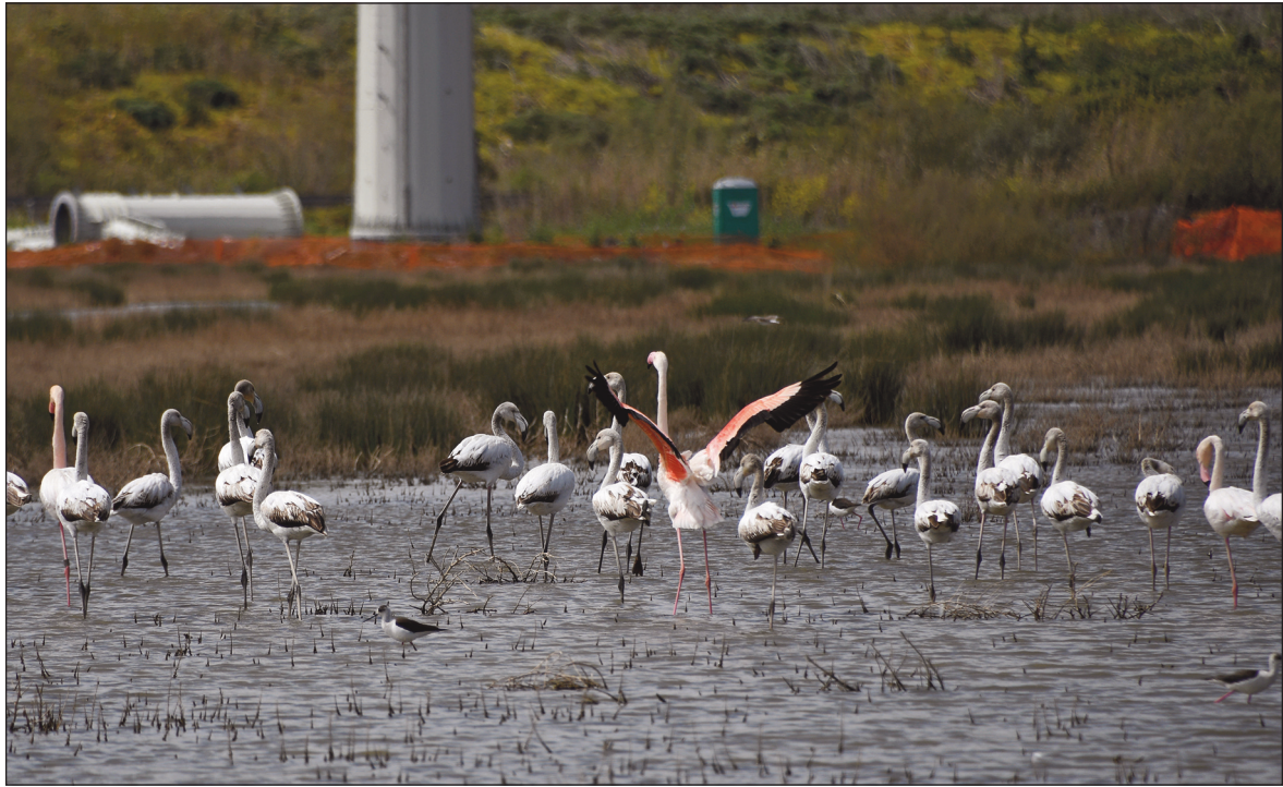
Figure 3. Greater Flamingo ( Phoenicopterus roseus ) and Black-winged Stilt ( Himantopus himantopus ) filmed during the construction of a support, which are stationed in an area that, when completed, will be topped by power line conductors (Lentini marsh, April 3, 2022).
